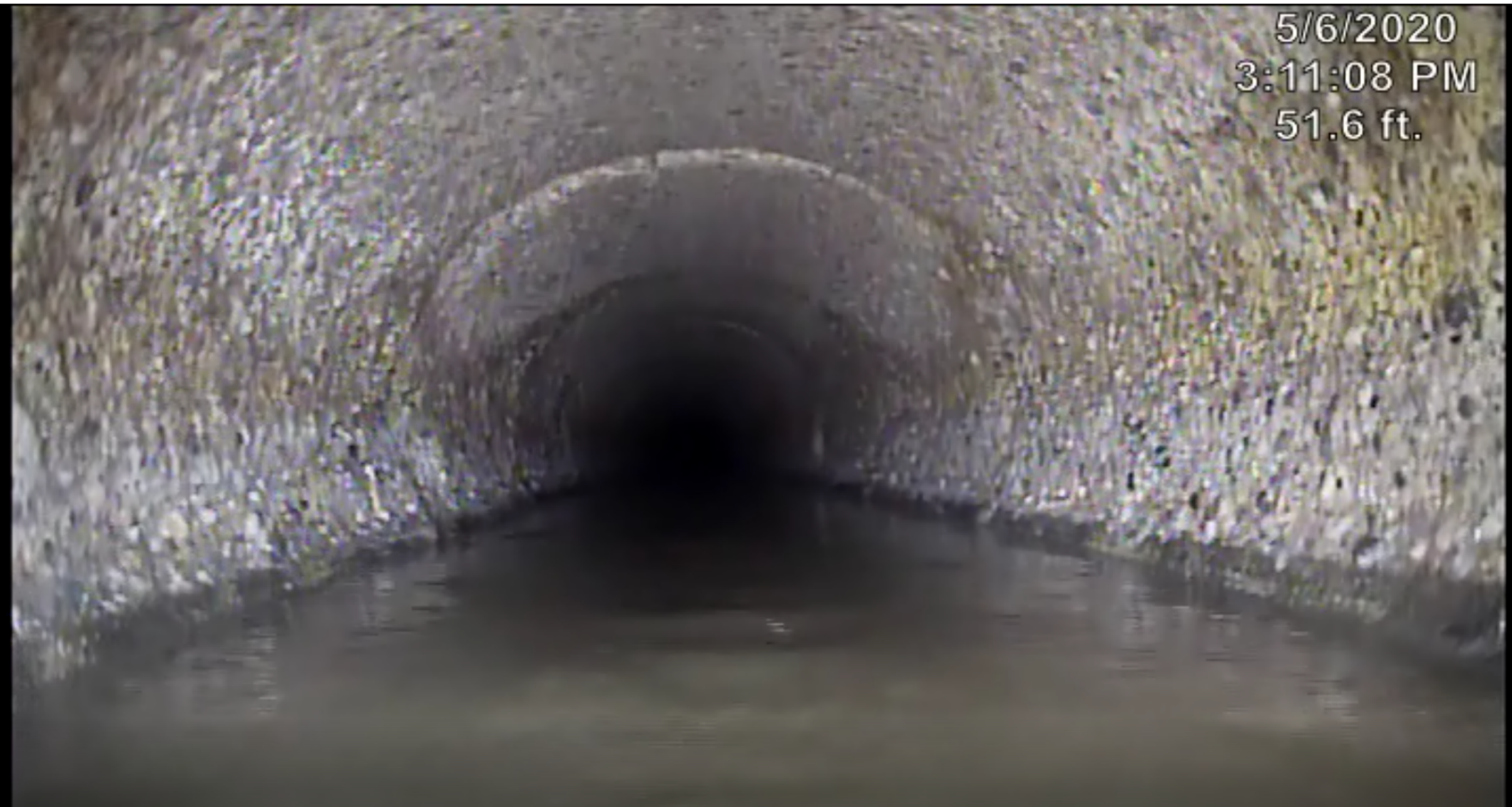
CITY OF SPARKS SANITARY SEWER CIPP LINING-Node '3520'-Node '3517'-
